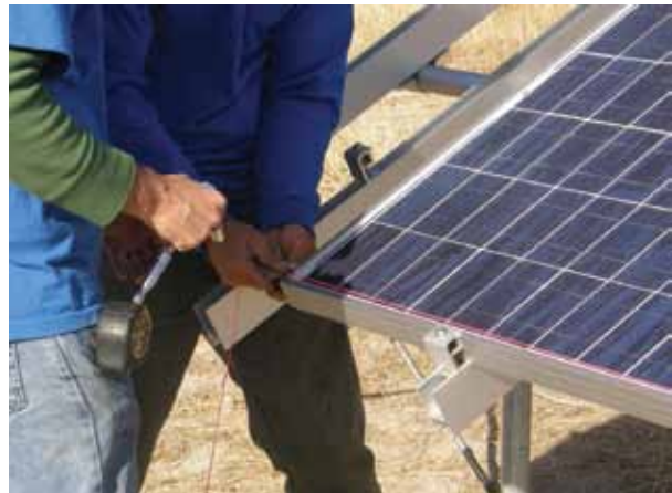
Aligning first row of modules
