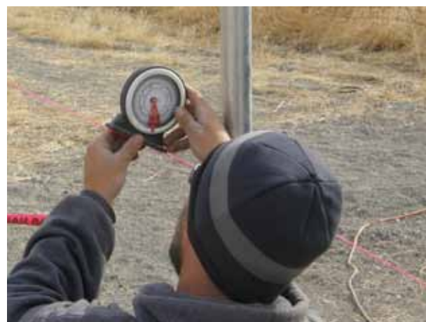
Check pipe frame levels
