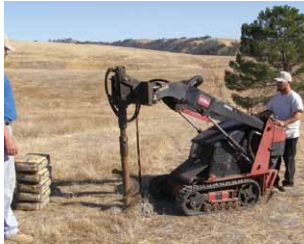
Digging holes with power auger
