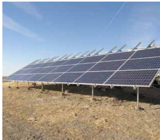
Three rows of modules installed
