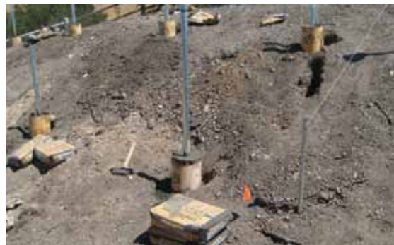
Poured concrete footings
