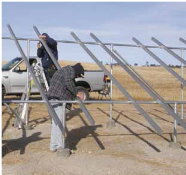
Attach rails to pipe frame
