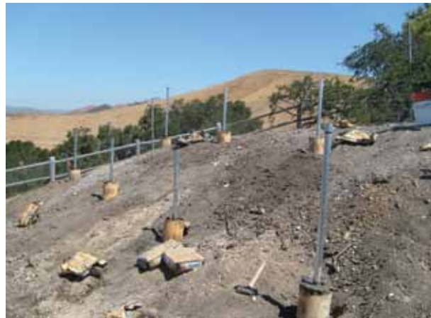
Install vertical pipes in concrete footings
