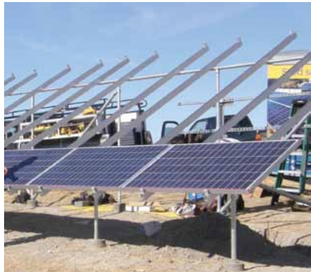
First row of modules installed
