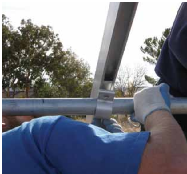
Attach rails using SnapNrack pipe clamps
