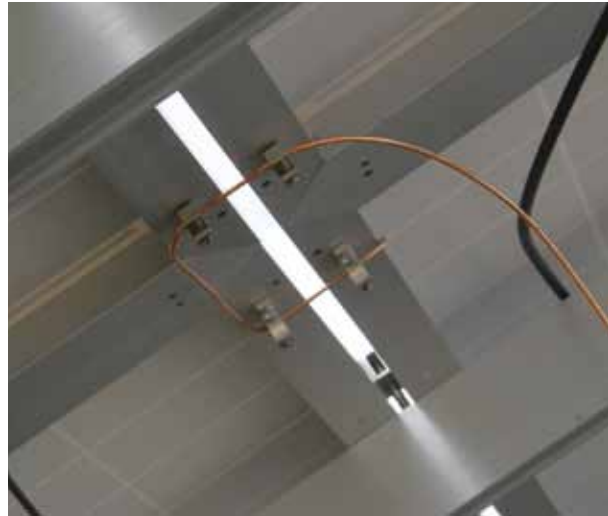
Grounding with lay-in style lugs
