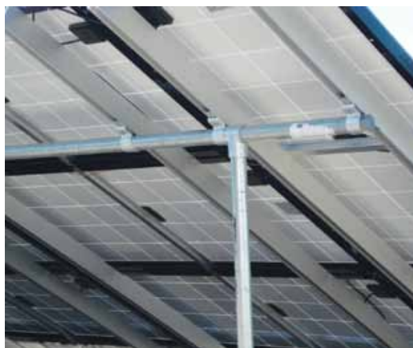
Check under the array for loose wires.
